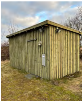
Den gamle pumpestation
